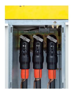
A separable mounting system ensures easy installation of the connector onto the bushing.
